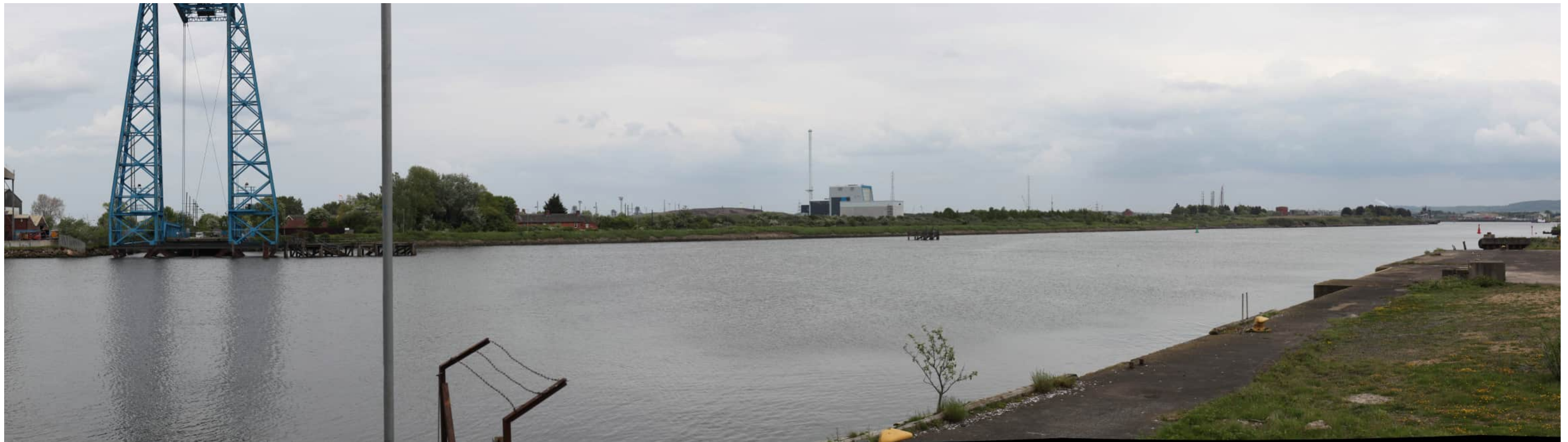
View 5: Transporter Bridge
